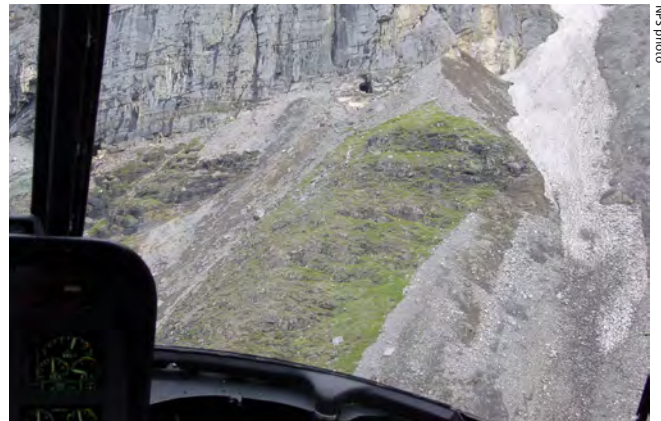
Figure 11. Helicopter survey of cliff adits.
