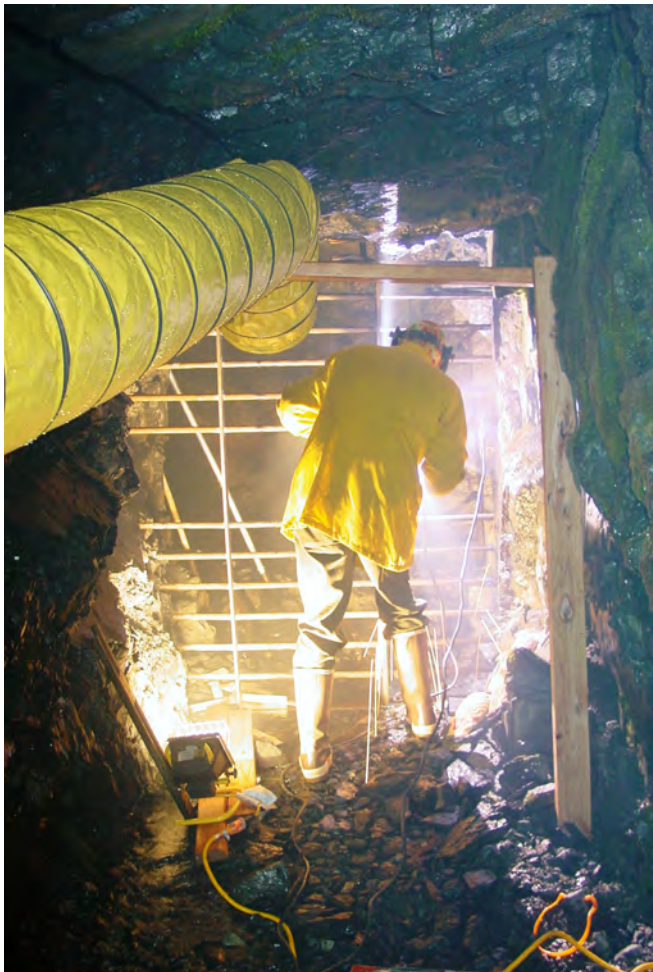
Figure 10. Welding a gate.
