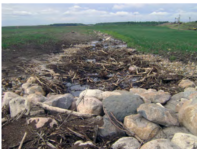
Figure 7. Drainage channel at Wapisiw Lookout (formerly Pond 1) at Suncor, July 2010.
