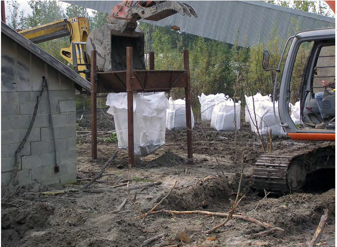
Figure 5. Removing super sacks of PCB-contaminated soils near Suntrana Creek in the Healy Valley.
