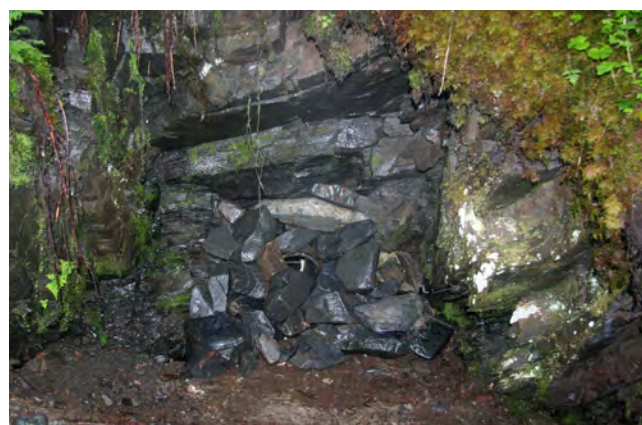
Figure 9. Polyurethane foam (PUF) closure with native materials.
