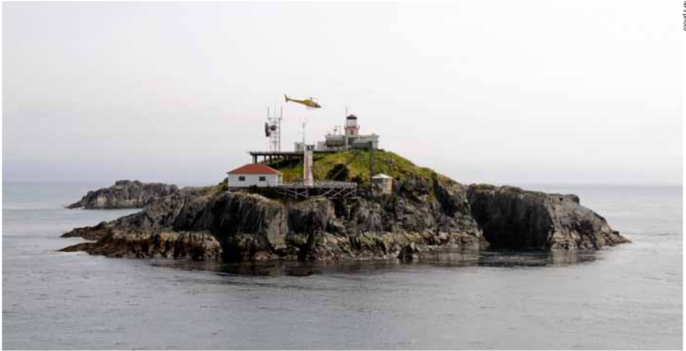
Figure 7. Cape Spencer Lighthouse is located within Glacier Bay’s wilderness. The station was constructed prior to wilderness designation and is managed by the U.S. Coast Guard. At least seven installations are co-located there, including a Federal Aviation Administration web camera, a National Weather Service weather station, a University of Alaska GPS station, and UNAVCO geodesy equipment.
